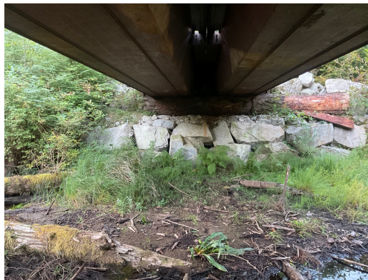
Left Bank Abutment when facing downstream
