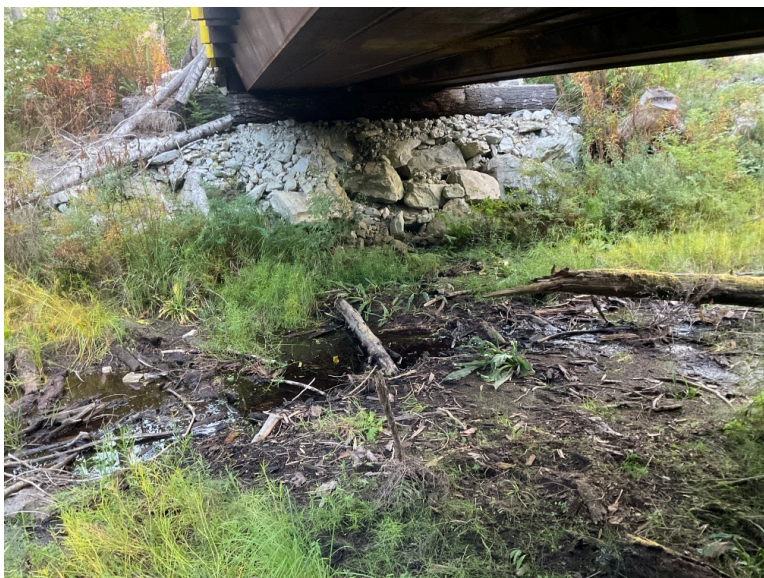
Right Bank Abutment when facing downstream
